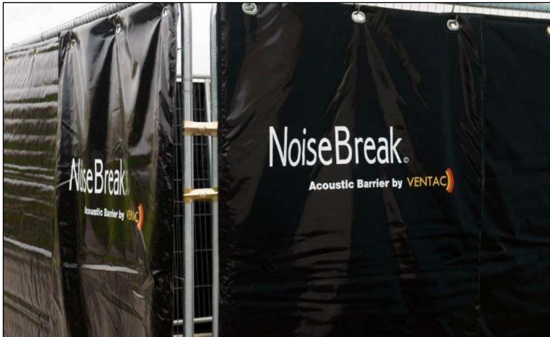
Figure 17.1: Temporary Construction Noise Barrier ©Ventac, extracted from Chapter 11 of this EIAR by Wave Dynamics.
